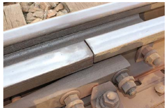
Fig.3 The heel of tongue rail
